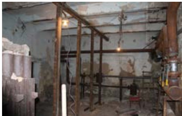
The basement of the city council in Kostyantynivka, Donetsk region, which was used by the IAG as an illegal prison. Photo by Volodymyr Shcherbachenko.
